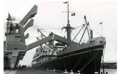
The meat loaders weighed 150 tonne and had about 250 pockets for transfer of meat from shed to ship's hold. In the hold each carcass automatically fell from pocket to a chute and at the end of the chute were watersides to manually stack each carcass in the hold. At full speed 2100 units could be transferred each hour.
